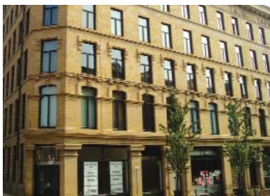
Broadgate House on Manor Row, a conversion into 89 residential units
