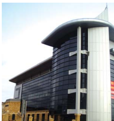
Shire House, Shipley, Airedale Road
